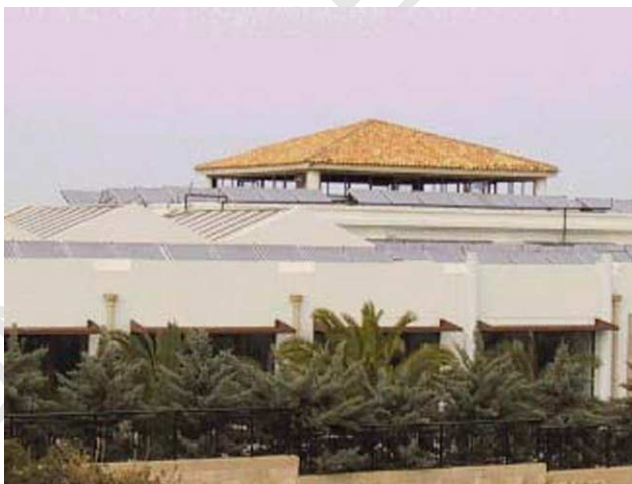
Fig. 6. View of Aldemar hotel complex.
