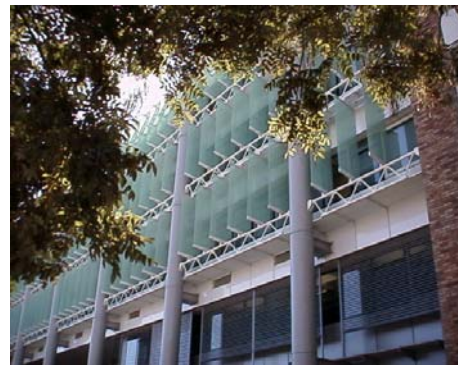
Picture 1 - AVAX Headquarters Building (front view)
